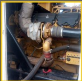
Power generator C32 2014, 12867h C32.GS, 3400V E Prime Power
